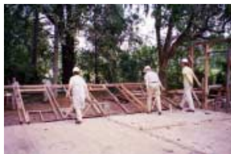
Figure 10 – Light-weight materials facilitate easy handling during deconstruction
