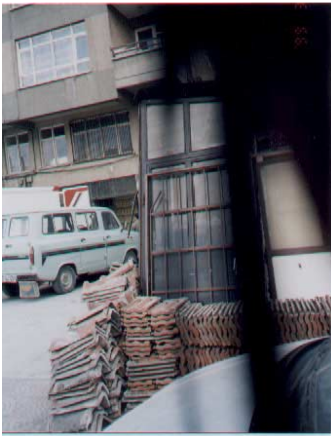
Figure 6. Roofing tiles from demolished buildings.
