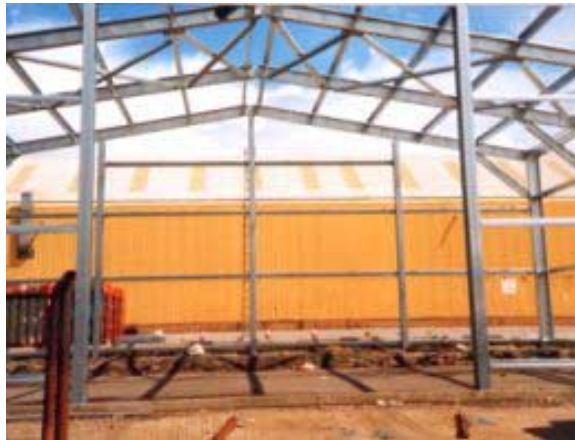
Figure 2 – Portals enable clear span solutions
