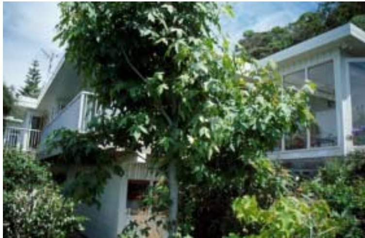
Fig 1 Lambie House east elevation, extensions are to north and south of central, remodeled upper floor centre and retained lower floor.
