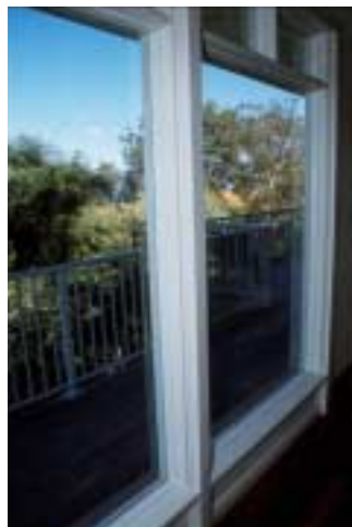
Fig 4 Retained existing window, interior view.
