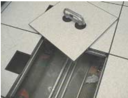
Figure 3 – Access floor seen from above
