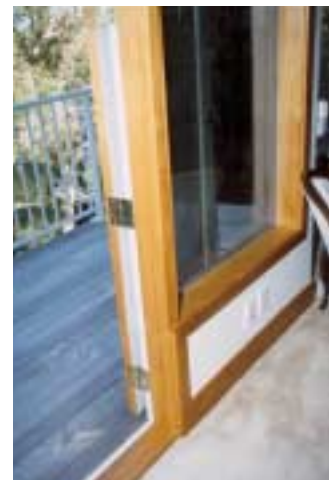
Fig 5 New window, interior view.
