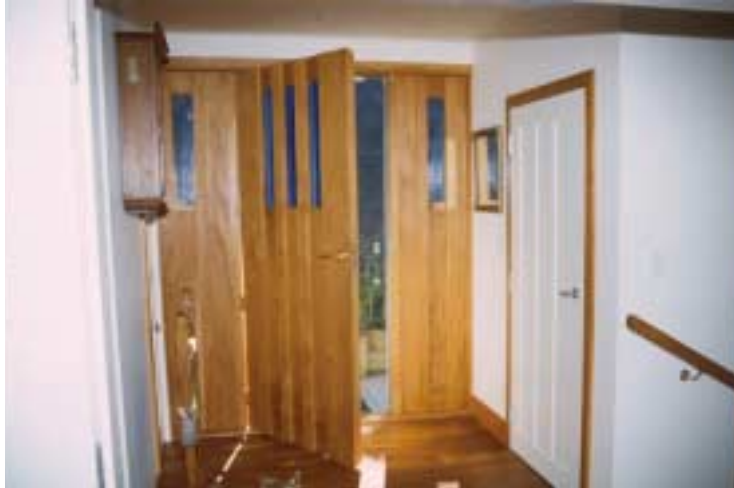
Fig 6 New entry door and reused flush door, paneled to give visual identity.
