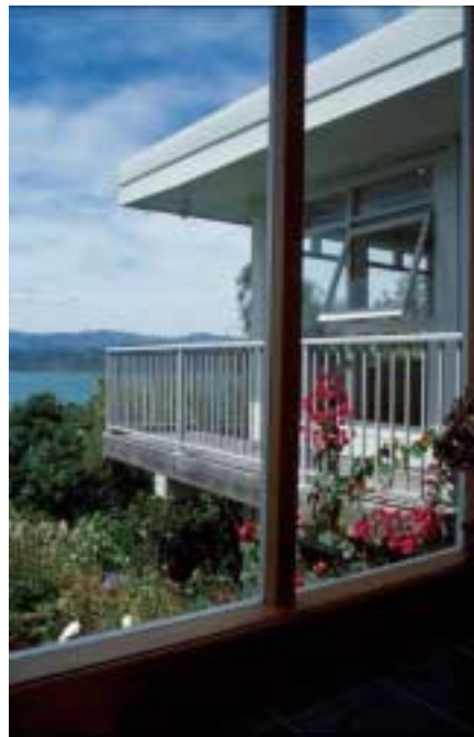
Fig 8 Thick roof edge resulting from encapsulating existing roof within new roof.
