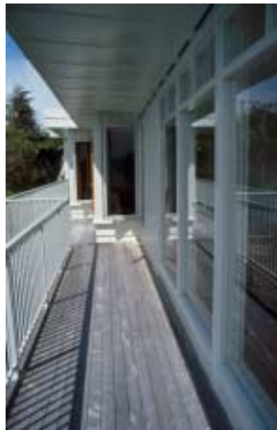
Fig 2 Visual integrity of reused windows, furthest away, new windows centre and retained existing windows, nearest to the camera.
