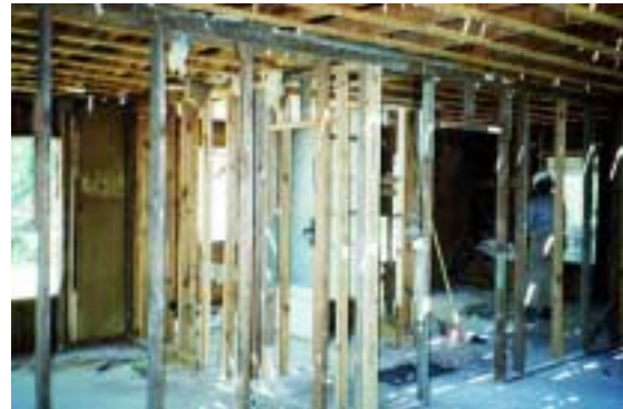
Figure 6 – Deconstruction of a regular dry wall system
