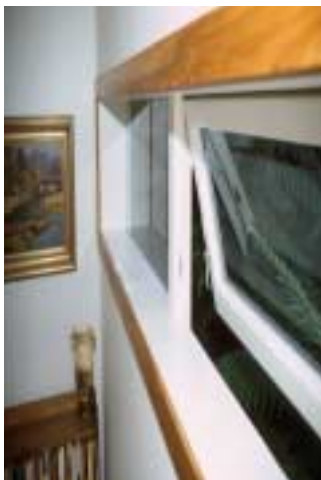
Fig 3 Reused window, interior view.
