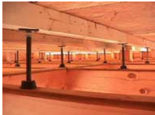
Figure 4 – Access floor seen from below
