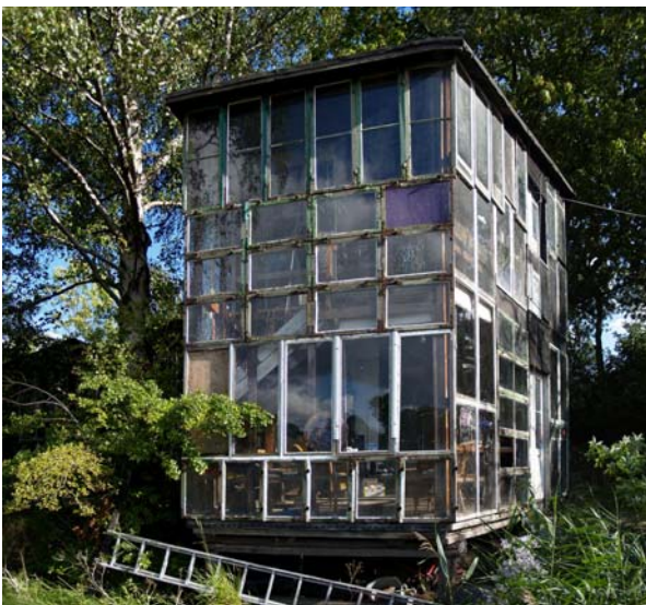
Figure 4. Glass House of window frames in Christiania, Denmark [11]
