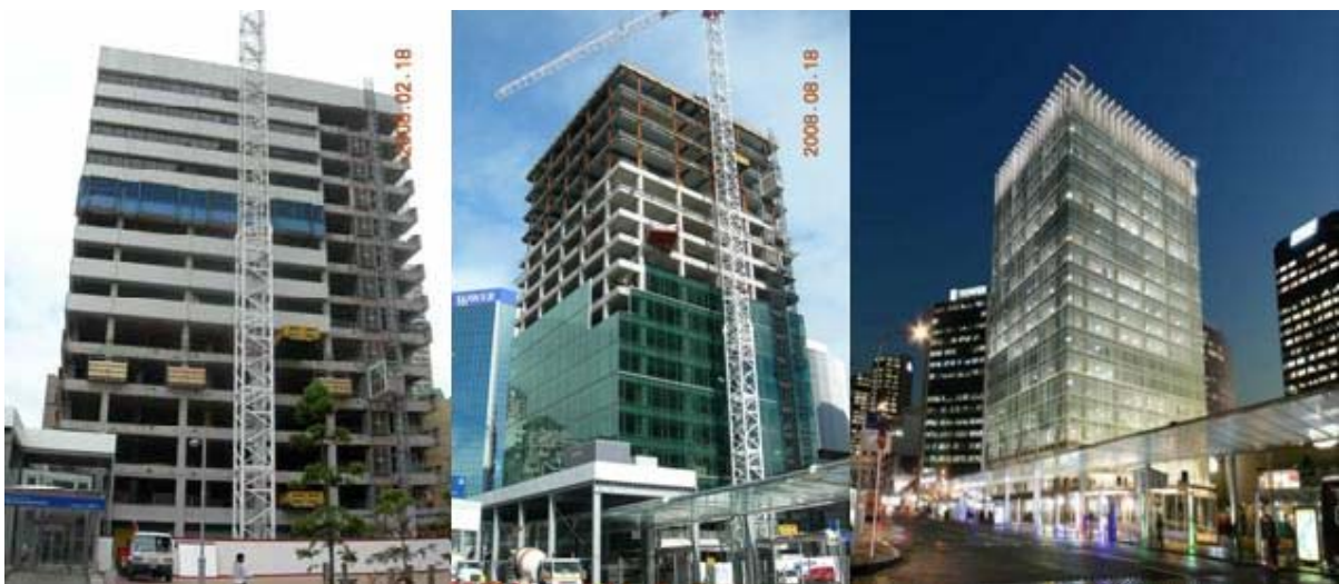
Figures 1, 2, 3 showing progressive removal of heavy concrete spandrel panels and their replacement with high performance double glazed unitised panels which allowed the addition of 4 new floors of accommodation. Note glazed pedestrian way at ground level that ties scheme into the city.
