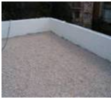
Fig.7. The insulated roof (photo Gil Peled)
