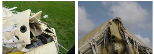
Figure 5: Errors in the connection of the fabric cover elements.
