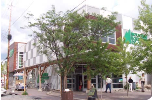
Figure 1: The Mountain Equipment Coop has pioneered component reuse in many of its retail stores. This one located in Ottawa reused many parts of the previous building on site, including the foundations.
