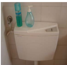
Fig.9. Installing water-saving fixtures (photo Gil Peled)
