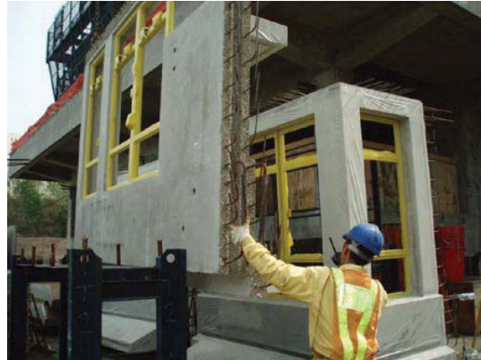
Figure 8. Prefabricated facade system
