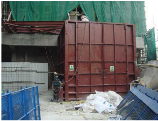
Figure 7. Refuse collection point at ground level
