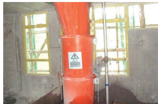
Figure 6. The refuse chute
