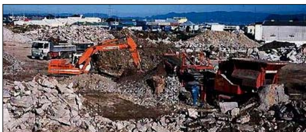
Figure 4 Impact Concrete Crusher from Ward Resource Recovery Ltd 51
