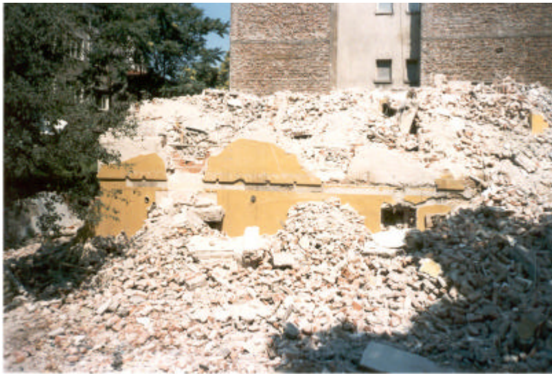
Figure 2 Rubble from the demolished building in a residential district of Ankara, has been left behind on the site.
