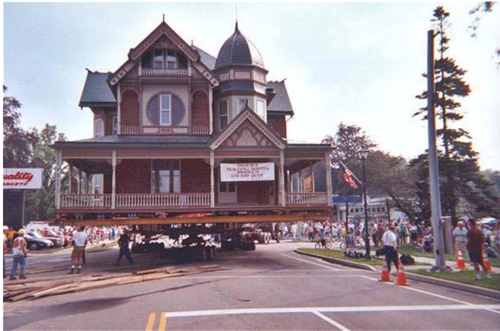
Figure 3. Moving an entire building to preserve its historical/architectural value
