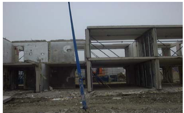
Fig5: After removing the floor it is clearly to see that the wall is not standing 90°. This will be fixed during construction
