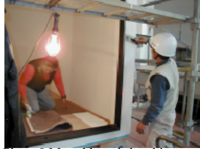
Photo 9 Mortar based sheathing (right) and non-skid rubber (left).
