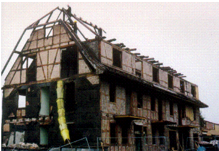
Dismantling of the Hotel Post in Dobel
