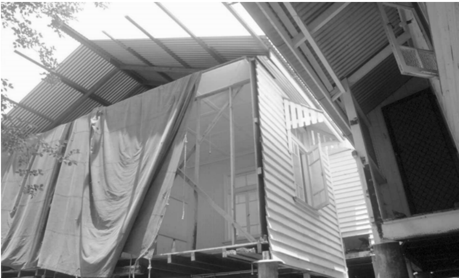
Figure 4 House during relocation – house has been relocated in two halves that are set apart to create new relationship (by Jeremy Salmon Architect).
