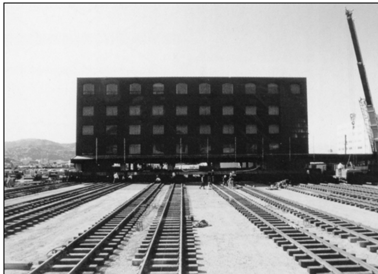
Figure 8 Reinforced concrete hotel being moved on its railway carriage
