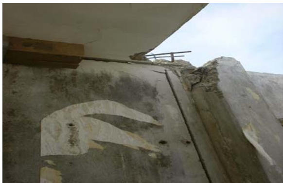
Fig 4: The newly settlement of the construction after sawing the wall in two sections. The right section will be removed.
