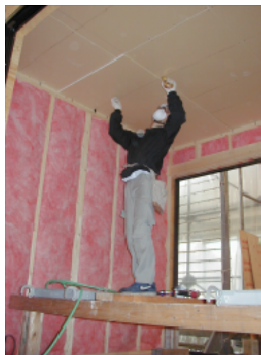
Photo 11 Ceiling gypsum boards hanged by metal connectors. Insulation fixed without using staples.
