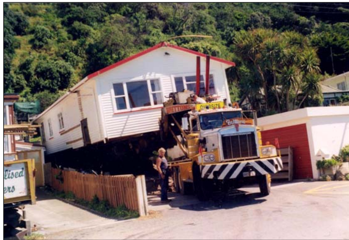
Figure 5 House leaving site on the back of a truck 69
