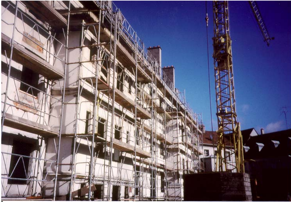
Figure 17 Dismantling in Mulhouse
