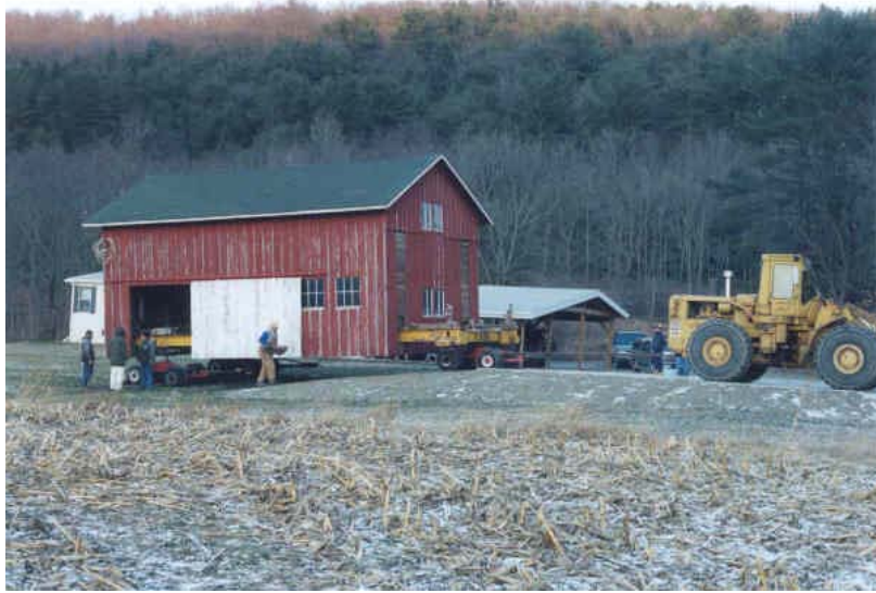
Figure 2. Relocation of a barn for adaptive building reuse
