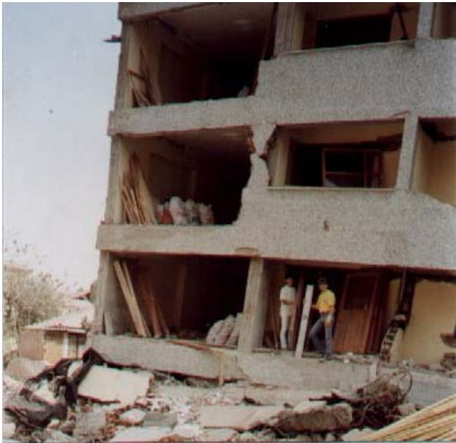
Figure 5: Recovery of building material from the severely damaged building in Figure 4; the structures beyond have been already been deconstructed and demolished [ij].
