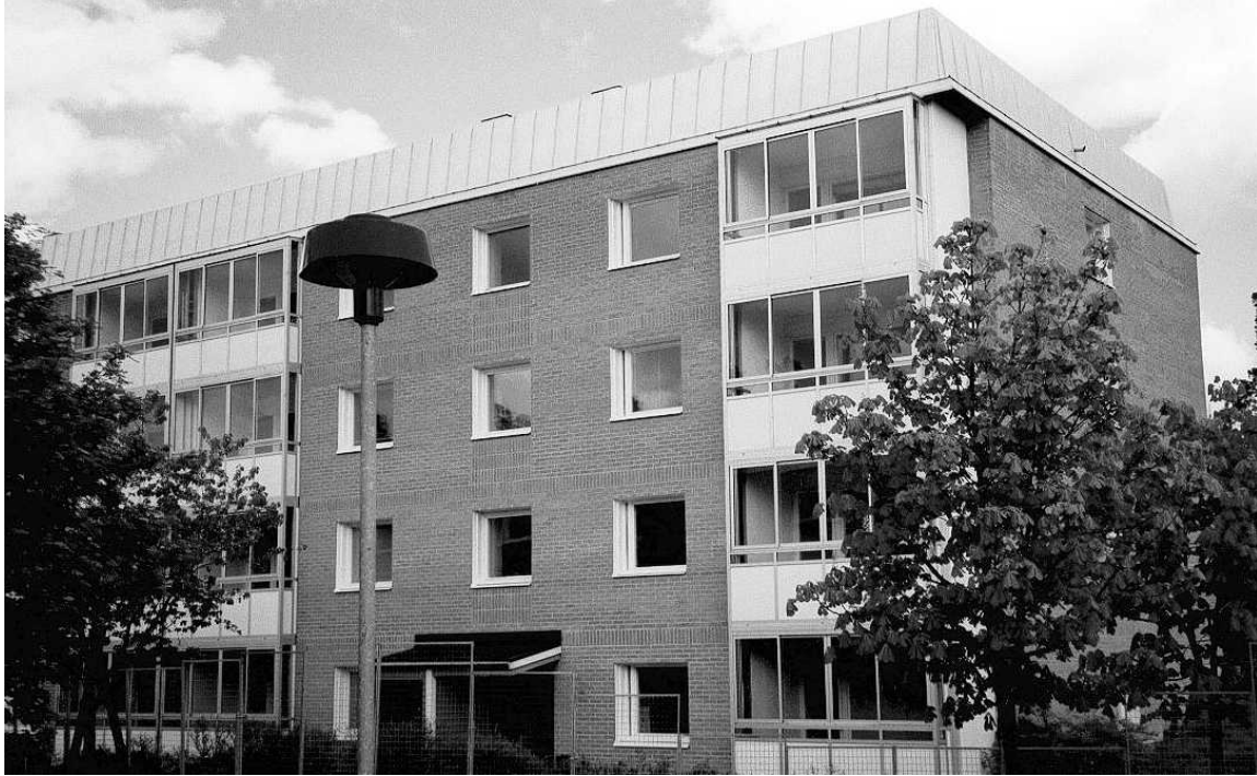
Figure 1. This is one of the apartment buildings in Finspång, Sweden that was torn down and functioned as a material source for a new building in Linköping, Sweden.
