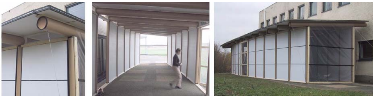
Figure 6: Pilot project – final assembly
