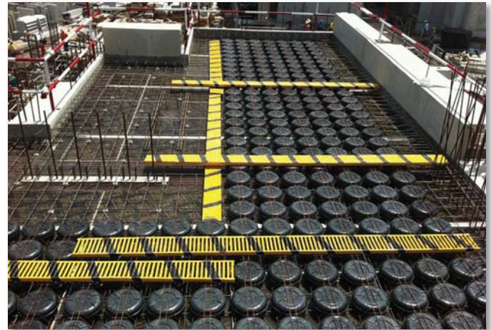
Pic.22 COBIAX WITH WALKING PLATFORM
