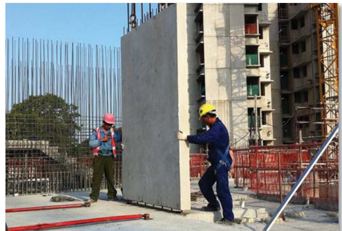
Pic.24 POSITIONING OF PRECAST WALL
