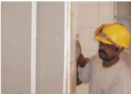
Pic.8.4 ARRANGE WALL TILES FOR FIXING WITH GLUE ADHESIVE
