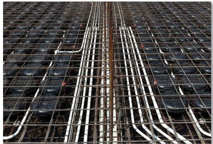
Pic.20 EMBEDDED M&E SERVICES WITHIN COBIAX VOID FORMERS
