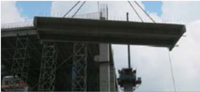
Pic.36 DOUBLE T-SLAB PRECAST BEING HOISTED UP FOR INSTALLATION
