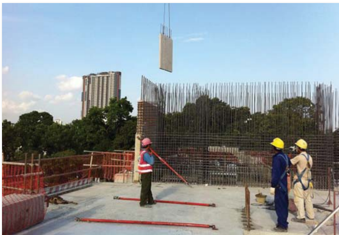
Pic.23 LIFTING OF PRECAST WALL
