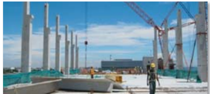
Pic.37 DOUBLE T-SLAB PRECAST BEING PLACED ONTO THE BEAM AND READY FOR REBARS INSTALLATIONS READY TO RECEIVE CONCRETE TOPPING UP
