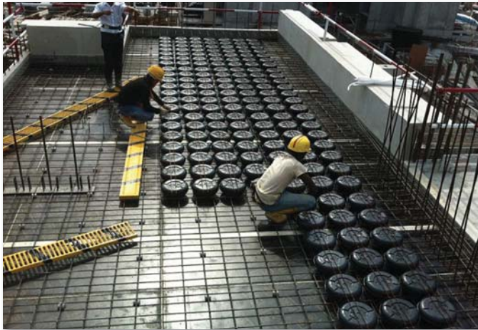
Pic.21 LAYING OF COBIAX IN PROGRESS
