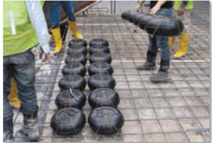
Pic.19 INSTALLATION OF COBIAX MODULES
