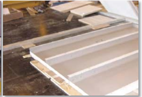
Pic.8.3 ARRANGE WALL TILES FOR FIXING WITH GLUE ADHESIVE
