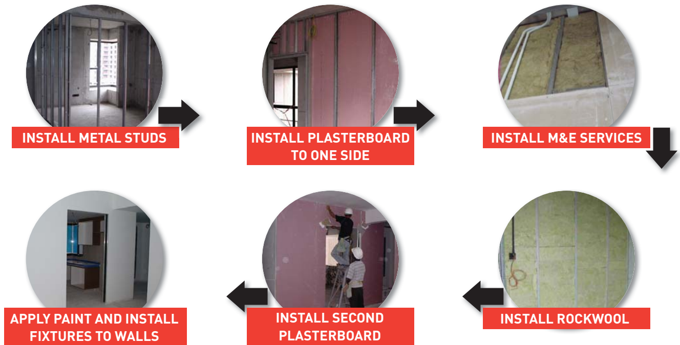
Pic.6 INSTALLATION PROCESS OF DRYWALL PARTITIONS
