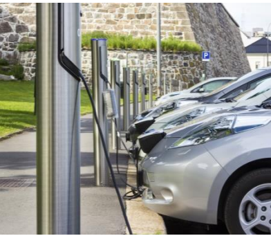
PRIVATE & PUBLIC EVSE ROLLOUT
